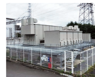
Installation of NAS battery system
