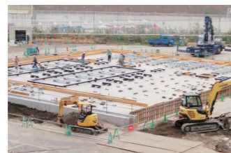
Construction of new substation
