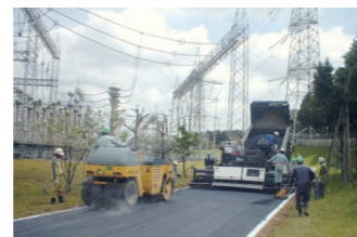
Paving road within substation premises
