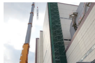
Installation of elevator for boiler building in thermal power plant
