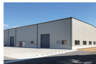
Construction of new spare parts warehouse
