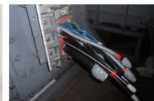
Waterproofing of cable penetration
