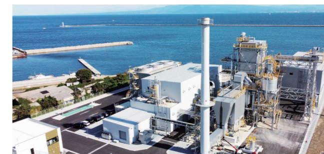
Sakaiminato Biomass Power Plant
