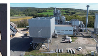
Abashiri Biomass Power Plant No. 2
