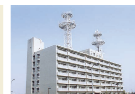
Electrical equipment at a public facility
