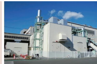
Civil engineering and construction of a gas engine cogeneration facility for a corporate client
