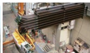
Repairing a boiler
