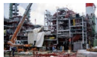
Installing a boiler in a chemical plant
