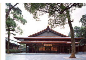
Electrical equipment for a special building
