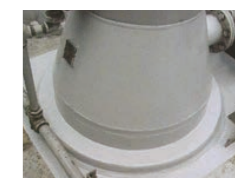
Repair of oil leaks from transformer bushing by chemical sealing
