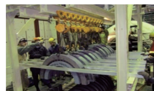
Multi-point support for ST diaphragm
