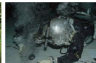
Underwater work in reactor containment vessels
