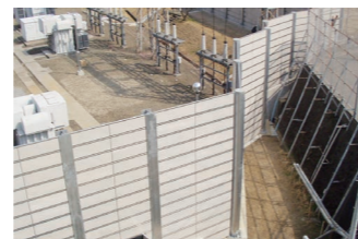
Construction of soundproof walls (H=7 m to 3.5 m, L=157.4 m)
