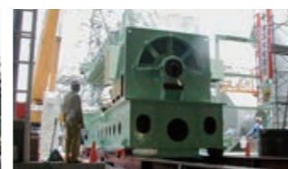
Installing a diesel generator
