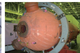
Disassembly, removal, and volume reduction of feed water heaters
