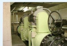
Micro hydro turbine (double type)
