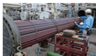
Overhauling a heat exchanger
