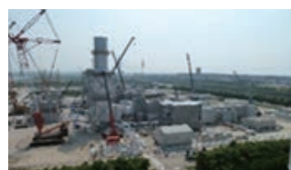
Construction of a thermal power plant
