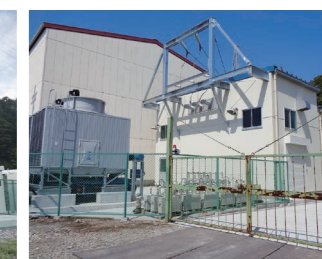
Construction of high-power testing facility
