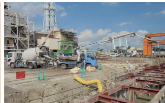
Construction of substation at thermal power plant
